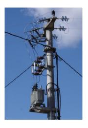
**Fig. 2.2:** Protection with fuses on the high-voltage side.
