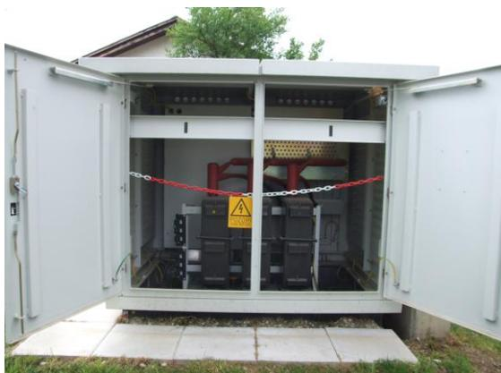
**Figure 12:** Example of fuse holder type VOH 2 with two type of voltage indication.
