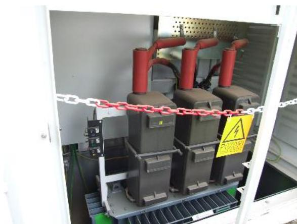
**Figure 8:** Fuse holder type VOH01 with connection Type C (EN5018), bolted T-plug, and mounted surge arresters
