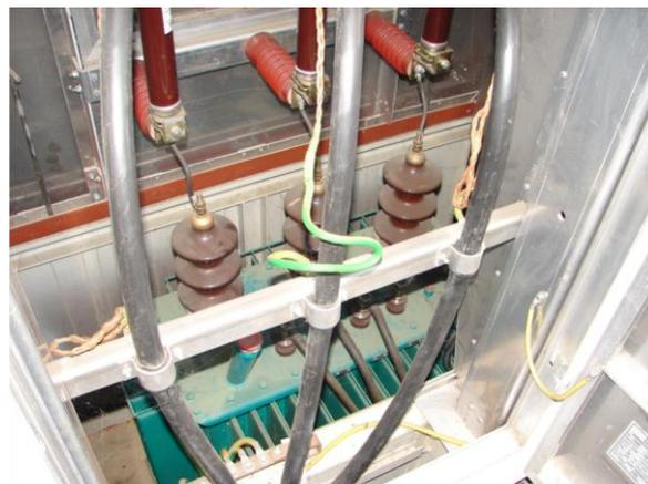
**Figure 13:** Example of not insulated places in a transformer substation
