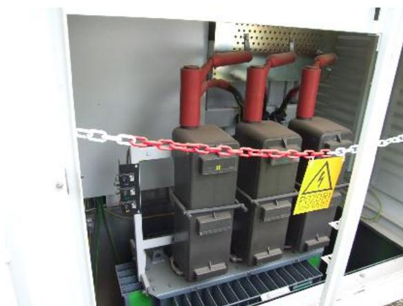
**Figure 14:** An example of application of fuse holder type VOH1, which insulates the HV part in a transformer substation
