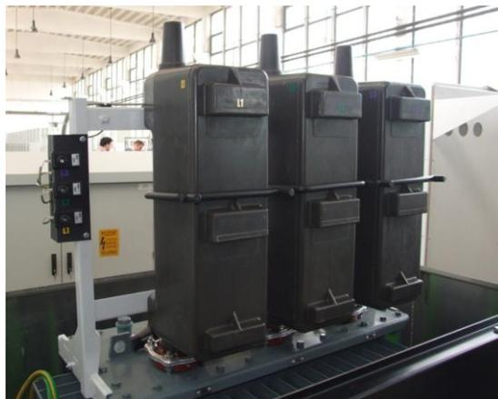
**Figure 1:** Insulated HV fuse holder VOH 01 (design by TSN) mounted on a transformer's cover (50 kVA).
