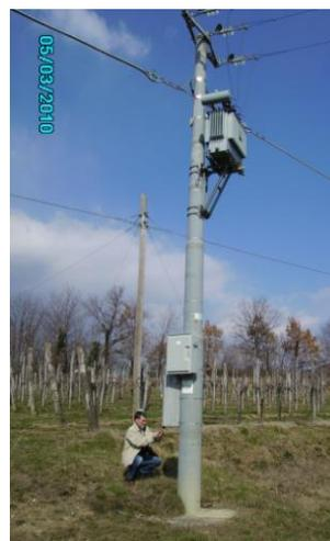
**Fig. 4.4:** Pole-mounted transformer substation with an unprotected transformer.
