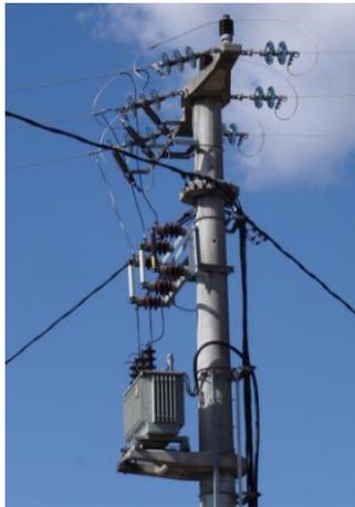
Fig. 2.2: Protection with fuses on the high-voltage side.
